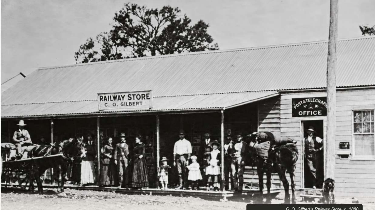
C. O. Gilbert's Railway Store, c. 1880 Morwell Historical Society reference - AI-assisted working restoration
